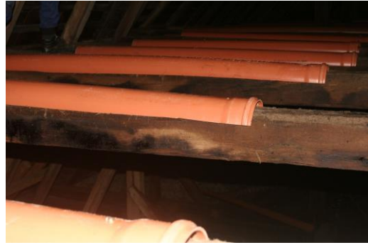
Picture C3-4: On the left - Cleaning timbers in church in Rajec; on the right – protecting timbers from guano by installing plastic tubes in church in Nemecká
