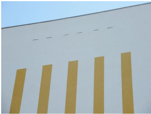
Picture C3-2: Bat boxes installed in thermal insulation
