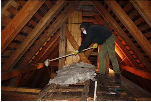
Picture C3-4: On the left - Cleaning timbers in church in Rajec; on the right – protecting timbers from guano by installing plastic tubes in church in Nemecká
