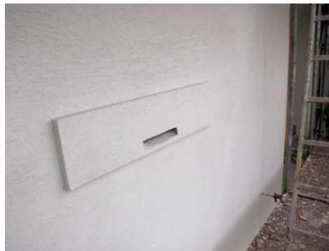
Picture C3-5: Special straight-through-hole batbox through which bats can access their original roosting sites in the crevices between panels
