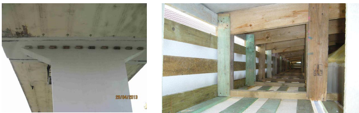
Picture C1-2: Swift boxes installed on road bridge in Malacky (left) and places for installation of boxes created in attics of a school in Žilina (right)
